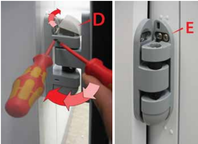
Pic. serie 13. Assembly of the hinges
